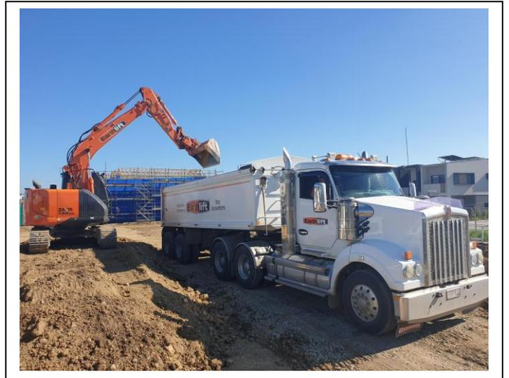
Before your projects start, whether that be a home, a commercial building, an industrial building, or any structure of this kind, you need to have the site cut. Site cutting means clearing a construction site from debris (vegetation, rocks) and perfectly levelling it with the use of some serious earthmoving equipment.
